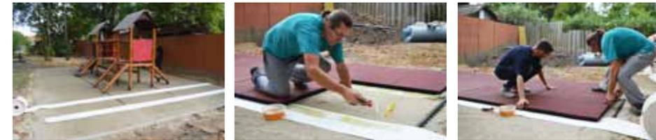
**5. THE INSTALLING STRIP:** Let's roll the strip upon the area (bright side upwards) in the entire length. Cut the strip at the ends of the area. With the help of a paint roller cover the strip by adhesive and place the rubber tiles upon. And repeat this process until the entire are is covered by tiles.
