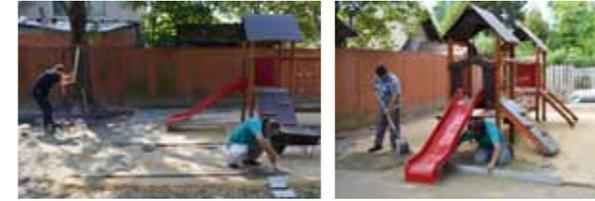
**4. MAKING OF GRAVEL BASE (UPPER LEVEL):** The 3 cm thick gravel base (is of 0-20 mm granules) should be compressed by vibrator and thus the basement will be hard enough for rubber tiles installment.
